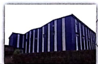
Liluah LED wires & Cables Unit
