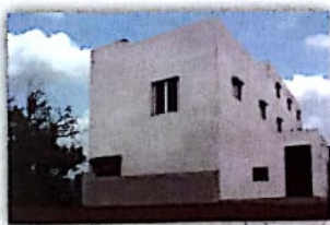
Baddi (HP) Switchgear Unit
